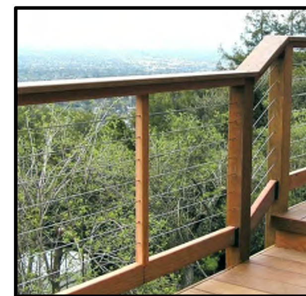
GUARD RAIL AT POOL AREA
