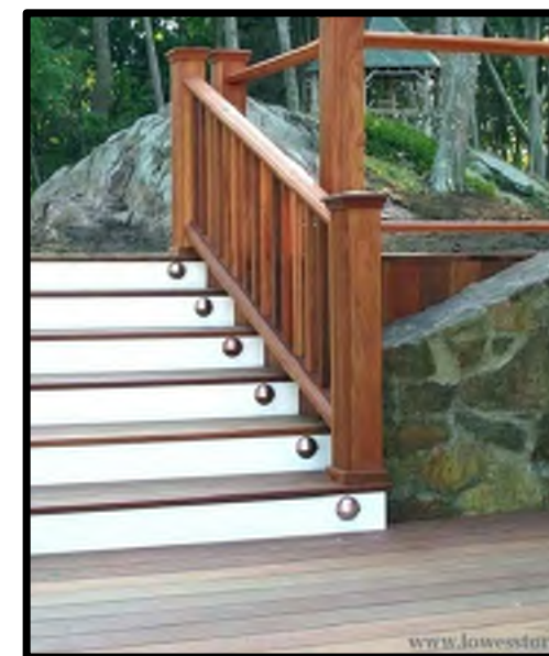
HANDRAIL AT STEPS
